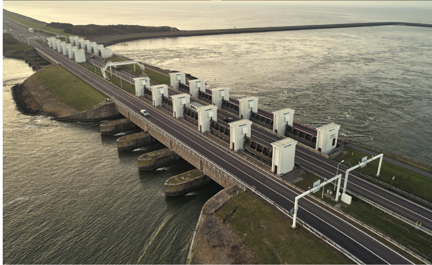
THIS PAGE AND OPPOSITE By day, the Netherlands' historic Afsluitdijk floodgates are unremarkable, but come nighttime they offer a futuristic experience. 'Without cars on the road, the structures do not illuminate,' says Dutch innovator Daan Roosegaarde of Gates of Light , his project that rejects energy-dependent lighting in favour of reflective material that emits light only when illuminated.
