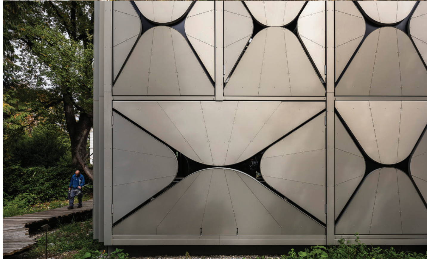
Shutters on the façade of a Swiss apartment building hydraulically open and close, creating balconies, overhangs and screens in turn. Architect Manuel Herz considered that it's how the building's residents choose to live, day or night, that will determine its appearance.
